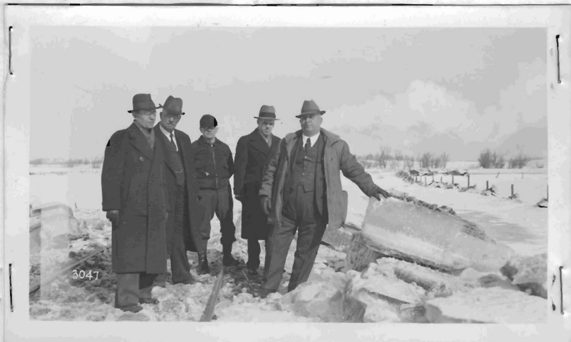
This pictures some of the operating officials that accompanied the heavy Duty Type A JORDAN with the high Plow on this job. Note the thickness of the ice which averaged from 1" to 23".
