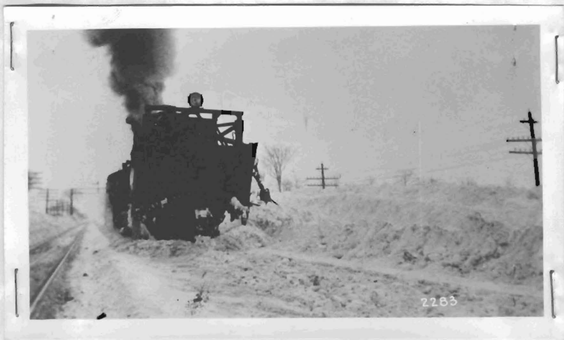
This is a companion picture of the preceding photograph showing the machine flanging the snow out of the adjacent track and also the left wing open, plowing the snow farther away from the main line. Note the adjacent track ready for travel.
