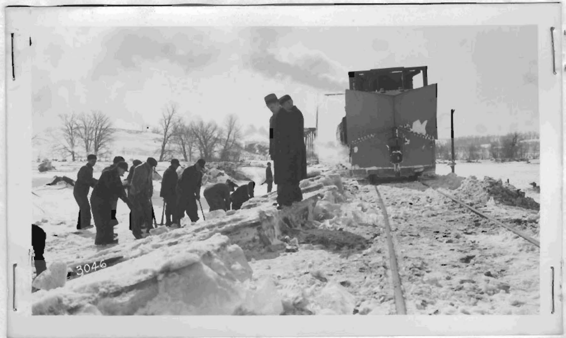
This view shows the track opened with the Type A Spreader-Ditcher and high front Snow Plow in the background.
