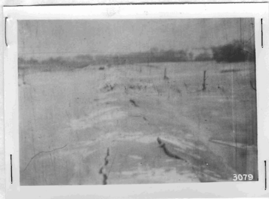
This view shows a railroad line which is covered with snow from 1" to 23" of ice above the rails. This condition was caused by an ice jam forming in an adjacent river, water backing up over the main line accompanied by a severe drop in temperature.
