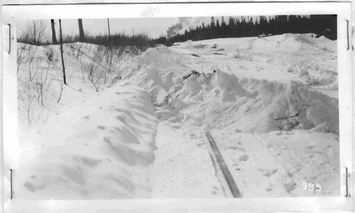
A view of a snow blocked line with the JORDAN Spreader equipped with the high detachable Snow Flow in the background.
