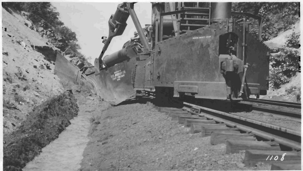
This view taken after one trip through with the JORDAN. Note the water preceding the machine down the track.
