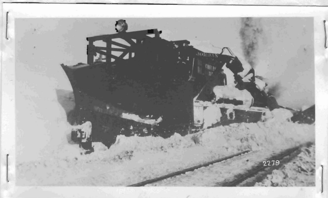
View showing a Type A equipped with high front Snow Plow flanging out one track, the left wing open and spreading the snow across the adjacent track while the right wing is plowing the snow out of the cut.
