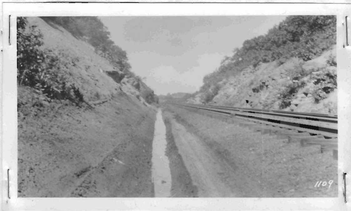
The finished job, showing the water draining out of the cut.
